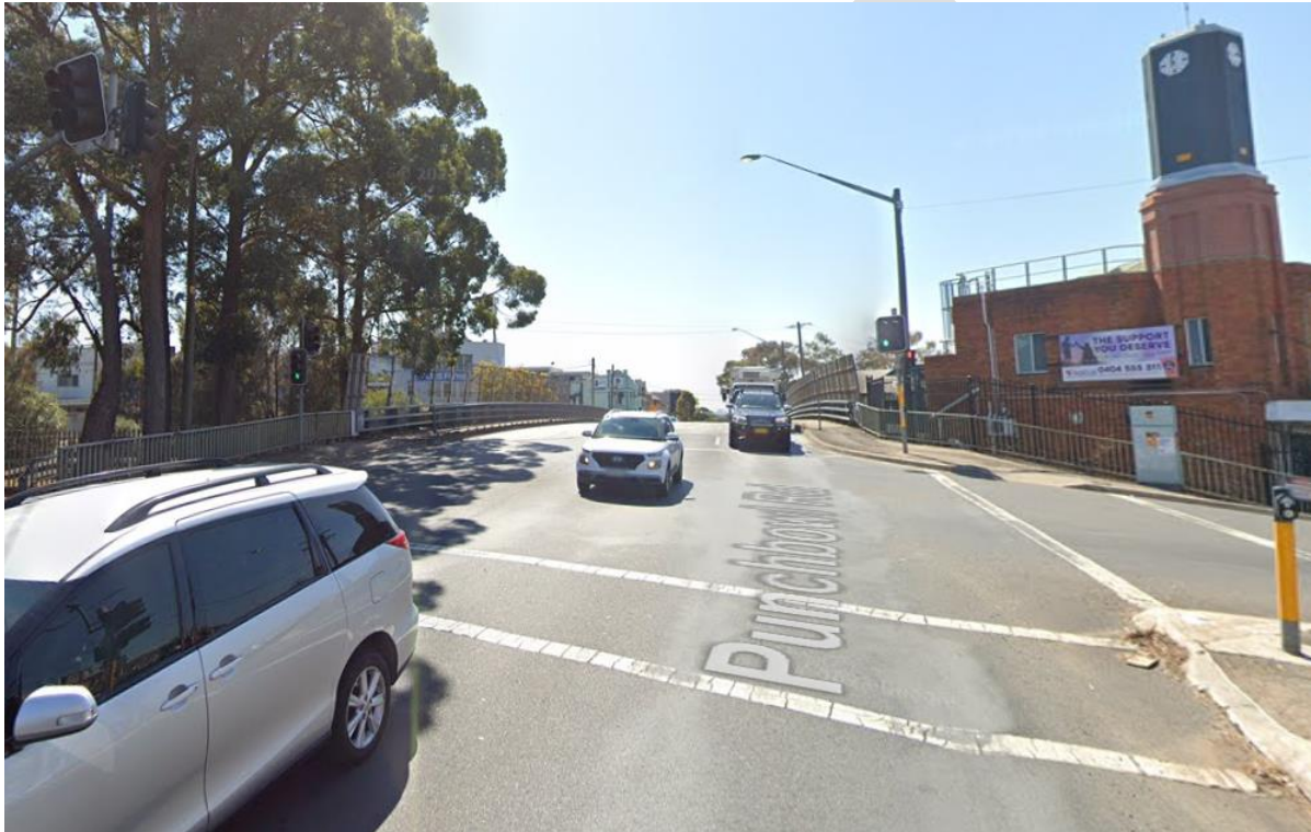
Figure 46: Punchbowl Road Bridge (Source: Google Maps)
