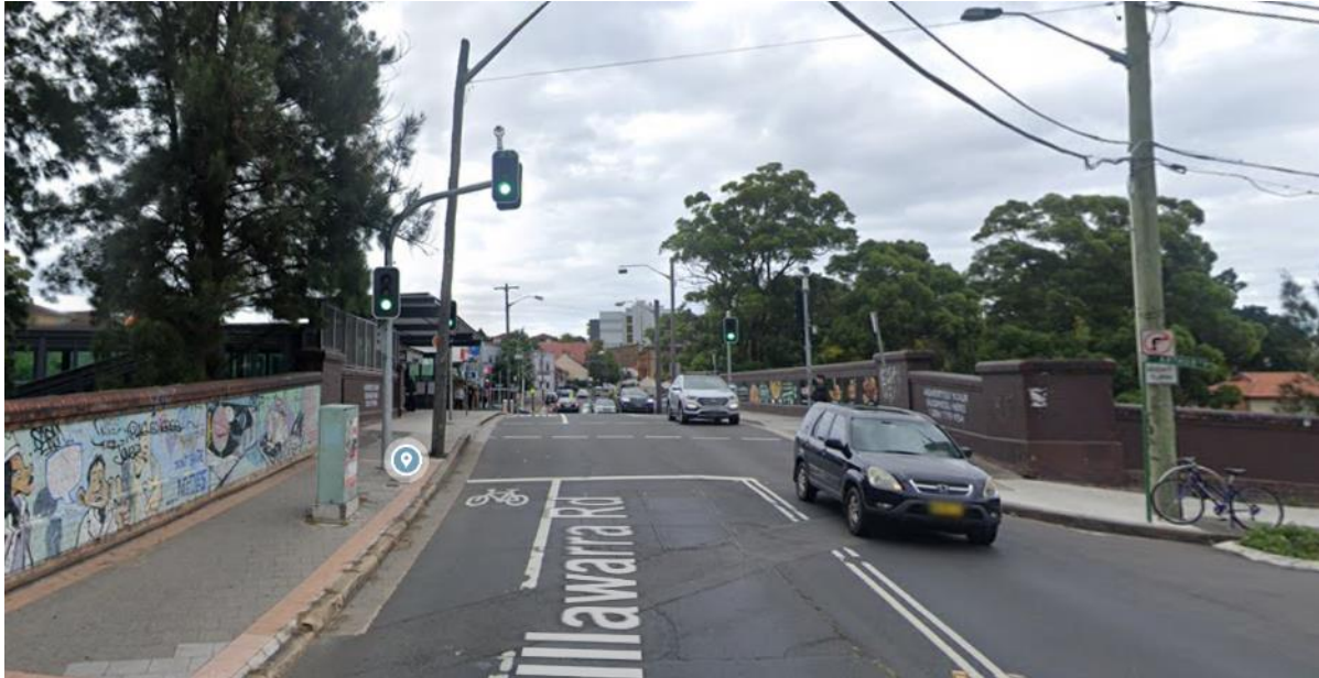
Figure 32: Illawarra Road Bridge (Source: Google maps)
