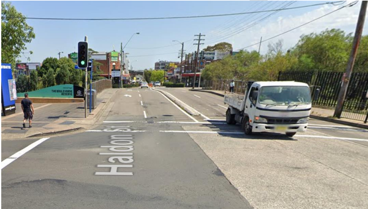
Figure 44: Haldon Street Bridge (Source: Google maps)
