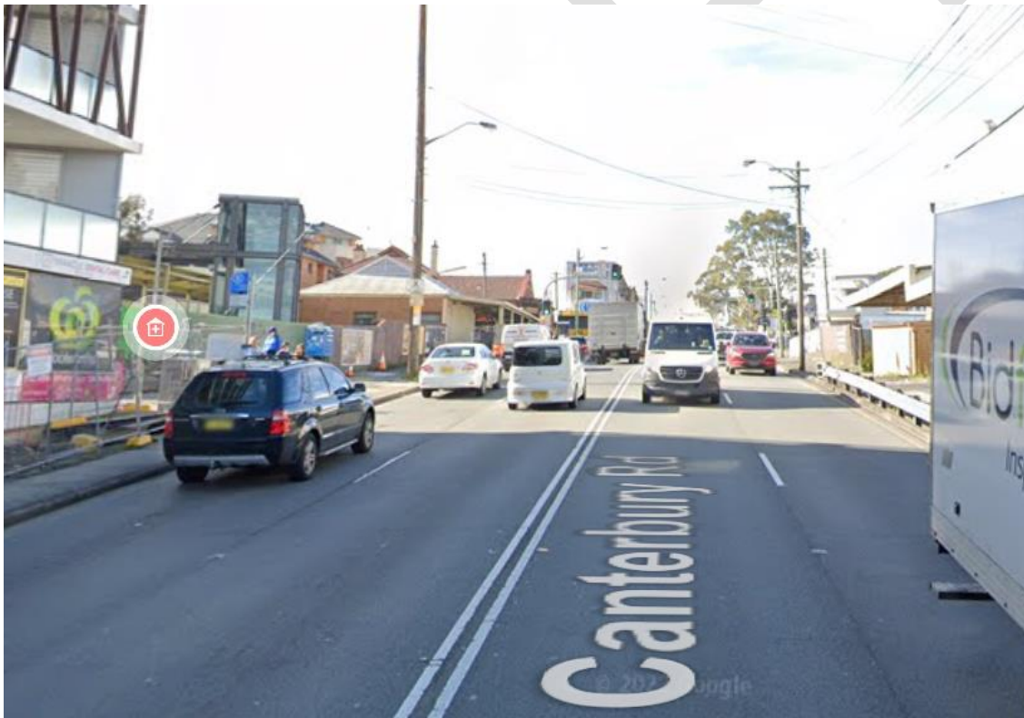
Figure 40: Canterbury Road Bridge (Source: Google maps)
