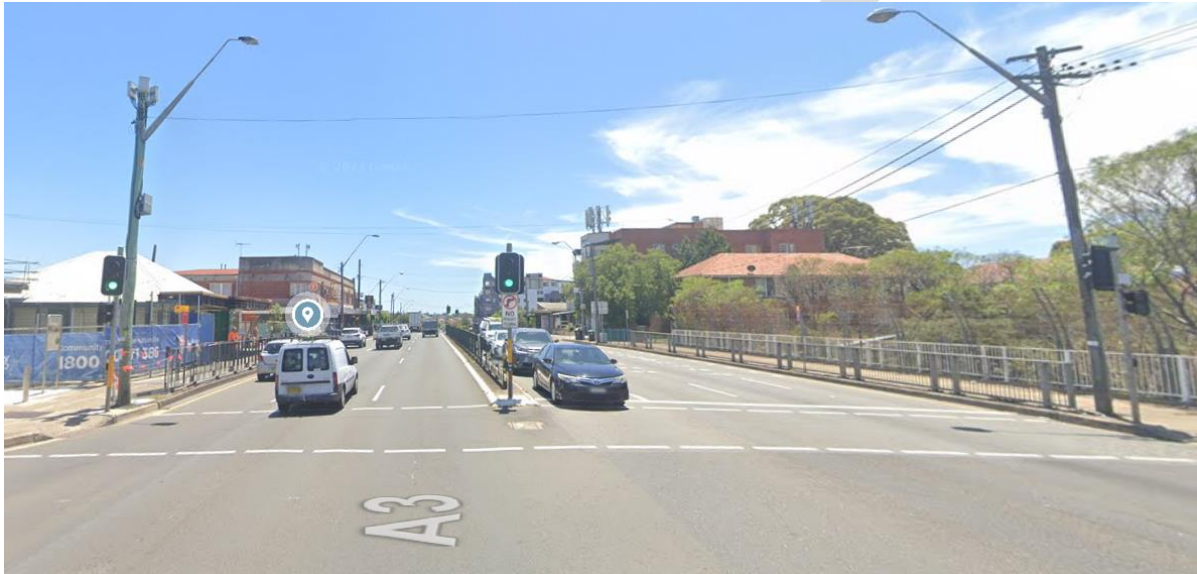
Figure 48: King Georges Road Bridge (Source: Google Maps)
